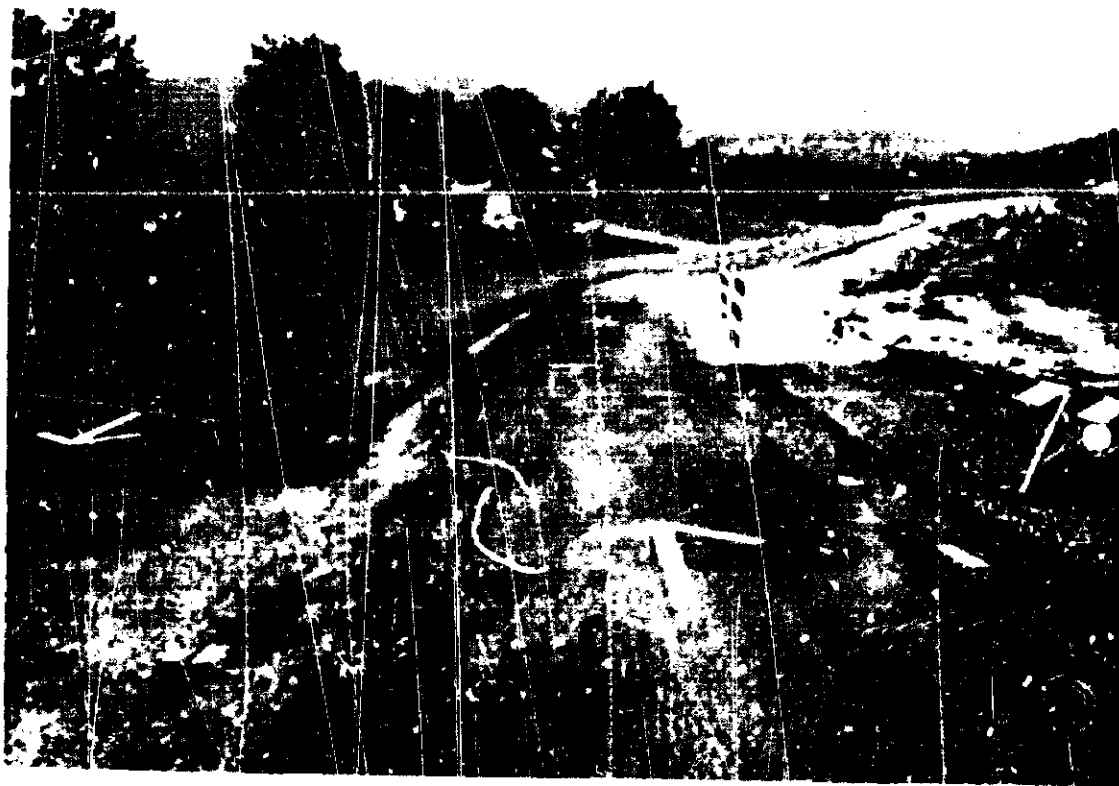
Figure 11.--Transition from existing alignment to new alignments. Pavement on right had been removed for construction of escape ramp.
